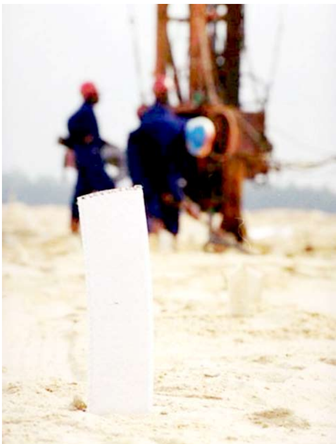
Detalhe do geodreno vertical (wick drain)
