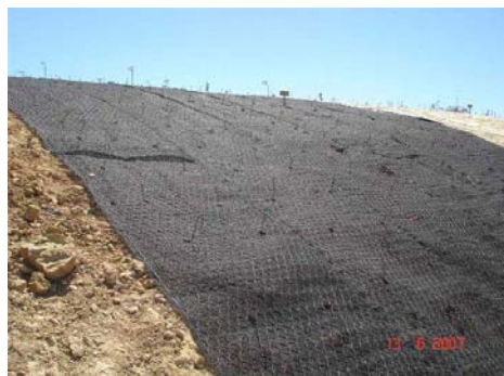
Figure 11. Geomat being unrolled in the slope Figure 12. Geocomposite protection installed in the slope
