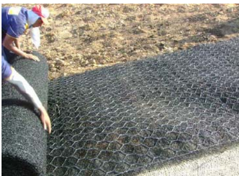
Figure 11. Geomat being unrolled in the slope Figure 12. Geocomposite protection installed in the slope
